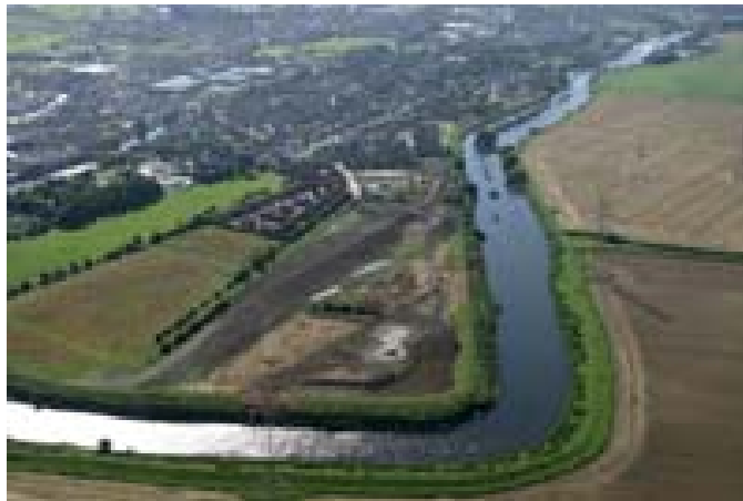
Figure 21: Project site, Knottingley Flood Alleviation Scheme
