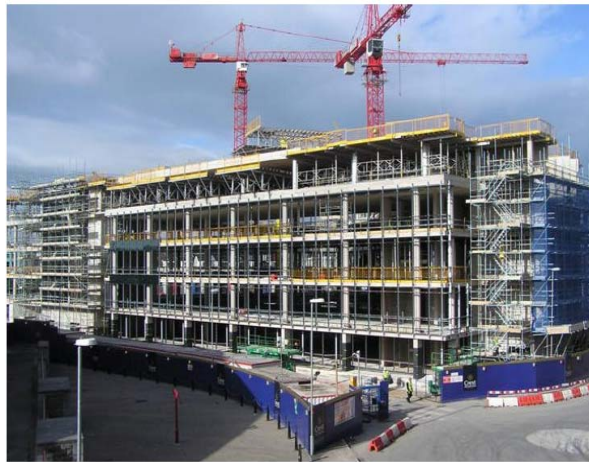
Figure 13: Construction site, Bristol Harbourside
