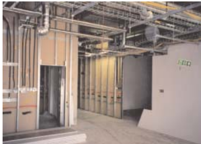
Figure 20: Pre-cut sheets in use in the internal construction of the hospital
