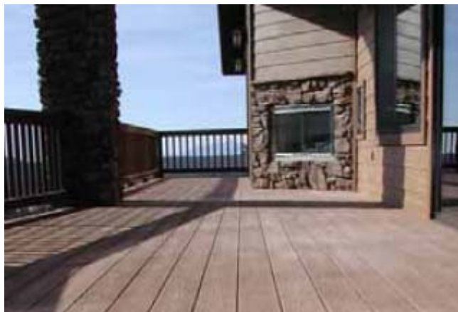
Figure 24: Plastic lumber deck
