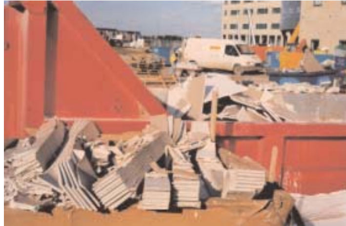
Figure 19: Plasterboard pallets used for delivery
